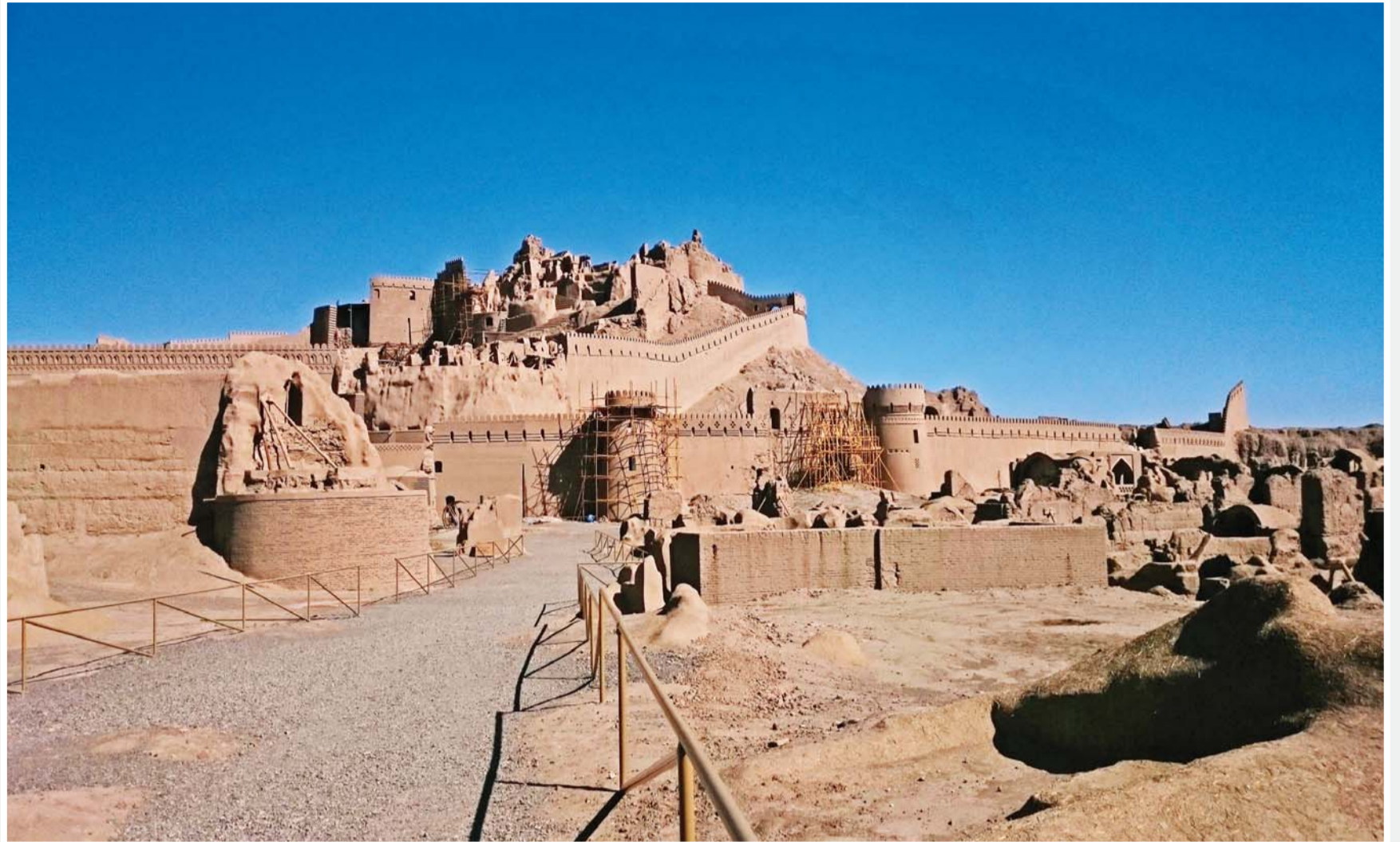
During the Parthian period the fort was expanded and became a citadel. At the end of the Parthian period, Arg-e Bam was captured by Ardashir I, the founder of the Sassanid Empire and they constructed new fortifications and walls.
