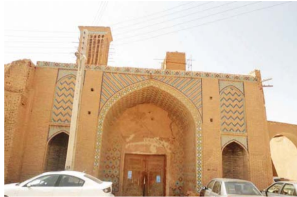
An exterior view of Vakil Caravansary in Kerman province
