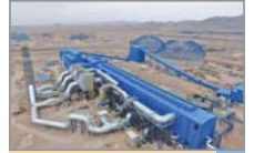
East Iran's first, biggest pelletizing unit becomes operational 4
