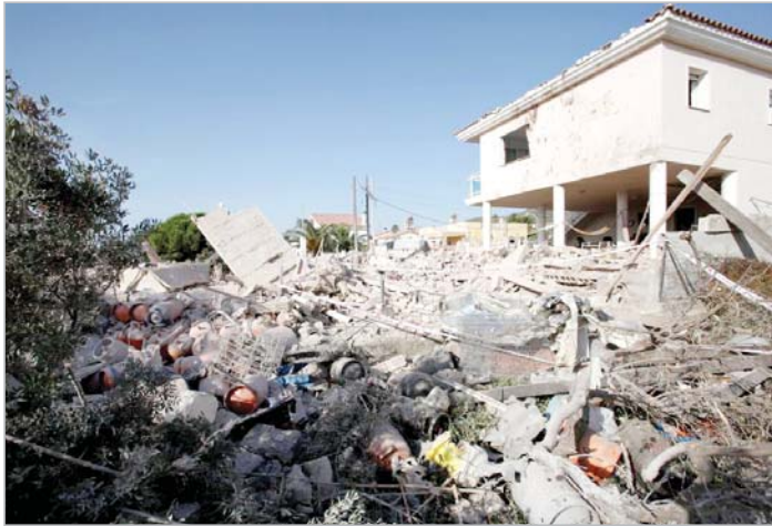
Police say the wrecked house in Alcanar is a focal point of the investigation.
