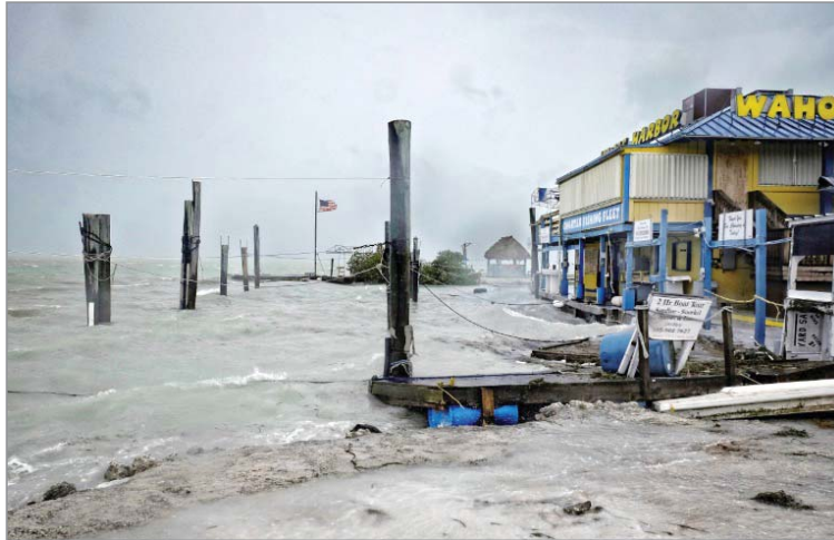
Rough surf churned up by the approaching hurricane damages the docks at Whale Harbour in the Florida Keys as winds and rain from the outer bands of Hurricane Irma arrive in Islamorada, Florida.
